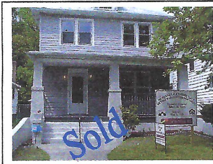
Rehab - 2711 Marshall Ave, NN 1520 sq ft, 2-story, 3 BR, 1.5 BA, large LR and DR, sturdy front porch, and detached garage.
