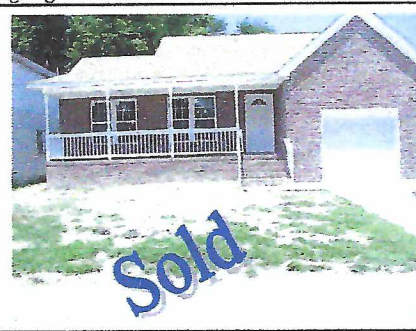
New Construction - 721 20 th St, NN 1366 sq ft rancher, 3 BR, 2 BA, Great Room, deck, covered front porch, and attached garage.
