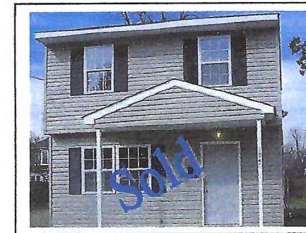
Rehab - 1047 29 th St, NN 1300 sq ft, 2-story, 3 BR, 1.5 BA, eat-in kitchen, LR, covered patio and driveway.
